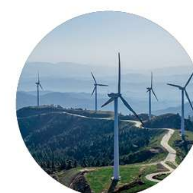
风力发电设备 Wind power plants
