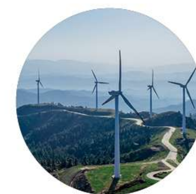
风力发电设备 Wind power plants
